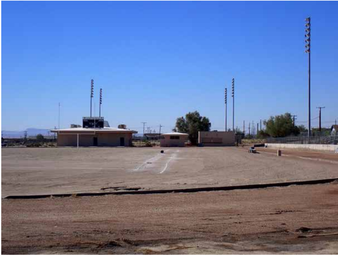
Trona High School Football Field (Photo Taken 09/05/2023)
